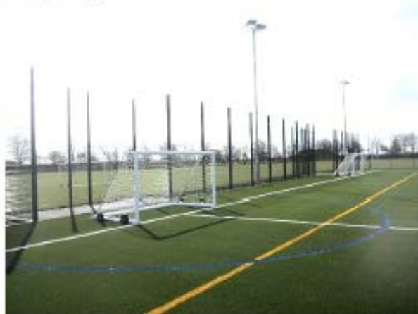
Typical 3G Artificial Grass Pitch (AGP) Installation
